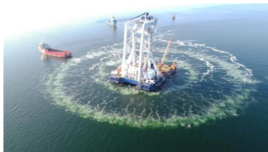
Bubble curtain used during construction.
